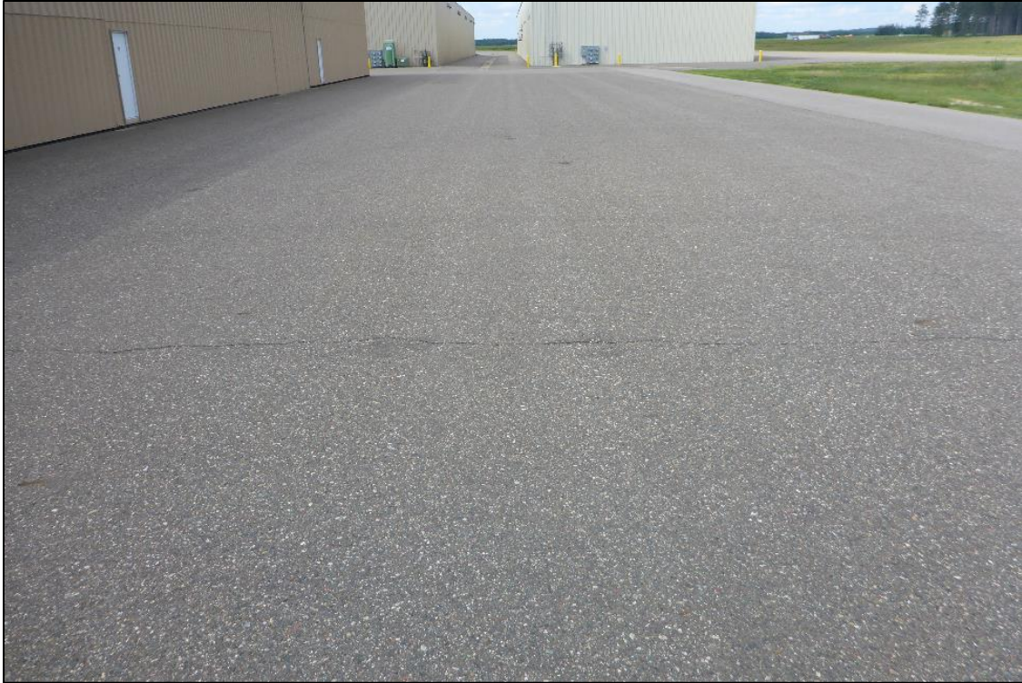
BRD TLA 001 (PCI = 100) – Pre-construction photo
